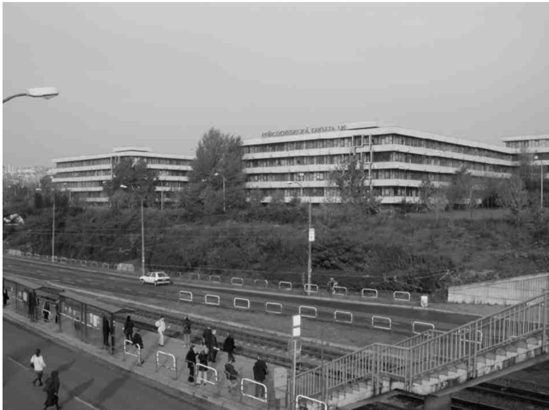
Photo 1. Faculty of Natural Sciences, Comenius University in Bratislava and the tram stop (west part)
