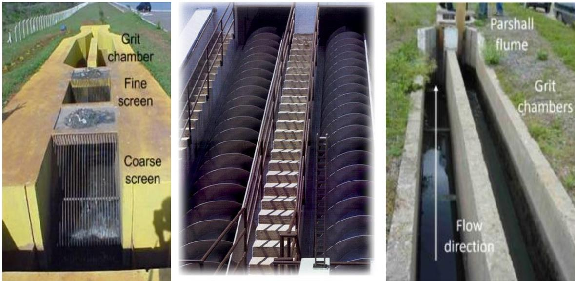
**Fig. 1.3.2. Manually-cleaned screens (left); sewage pumping into the next technology units of wastewater treatment plant (middle); horizontal flow grit chambers (right).**
