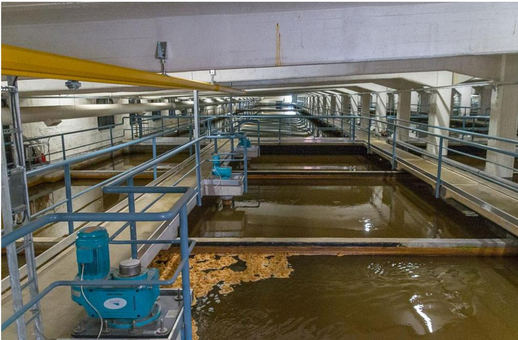
**Fig. 1.2.6. View of coagulation & flocculation process in real waterworks.**
