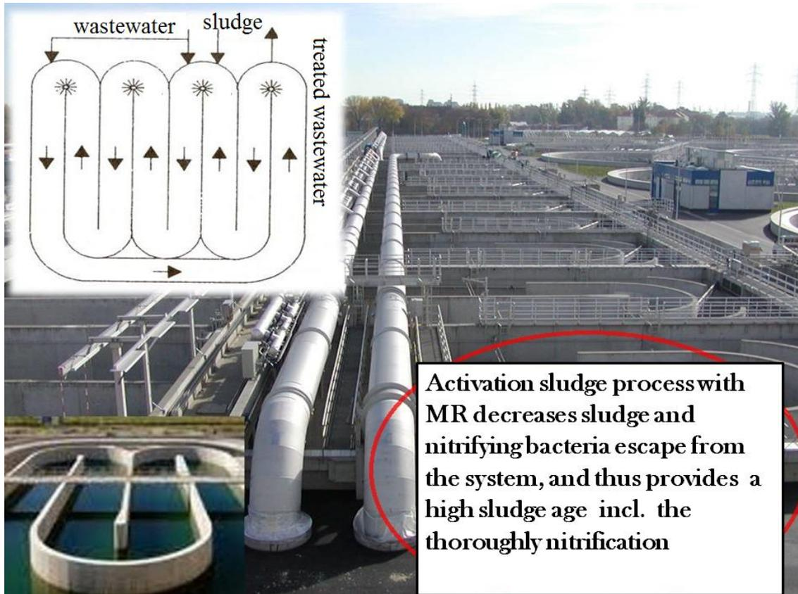
**Fig. 1.3.8. Carrousel system as the most simple arrangement for the carbonisation, nitrification and denitrification of wastewater in wastewater treatment plants.**
