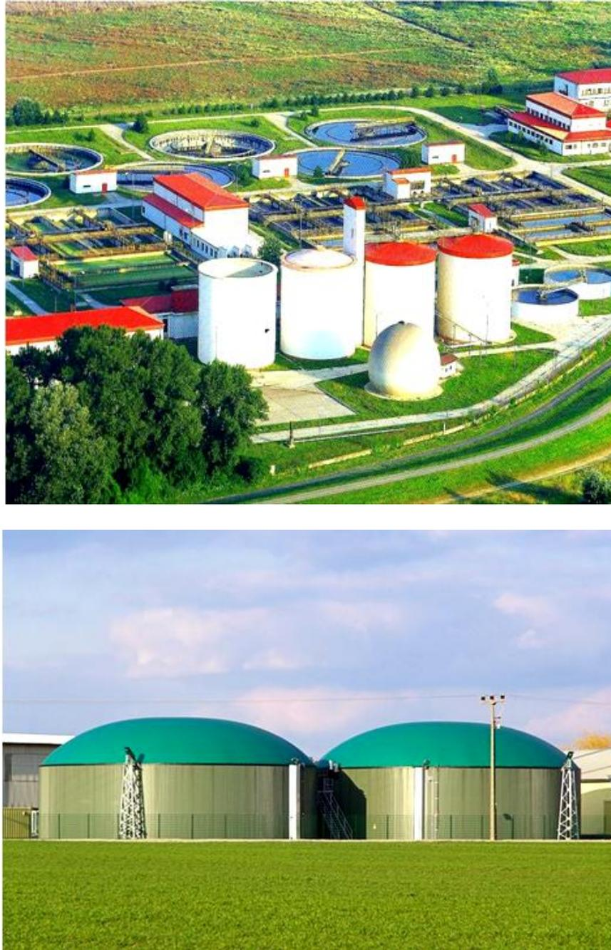
**Fig. 1.3.16. Anaerobic digestion towers (upper figure municipal wastewater treatment plant for the city residence Petržalka of Bratislava capital where biogas production during sludge digestion process is combined with electricity co-generation unit).**
