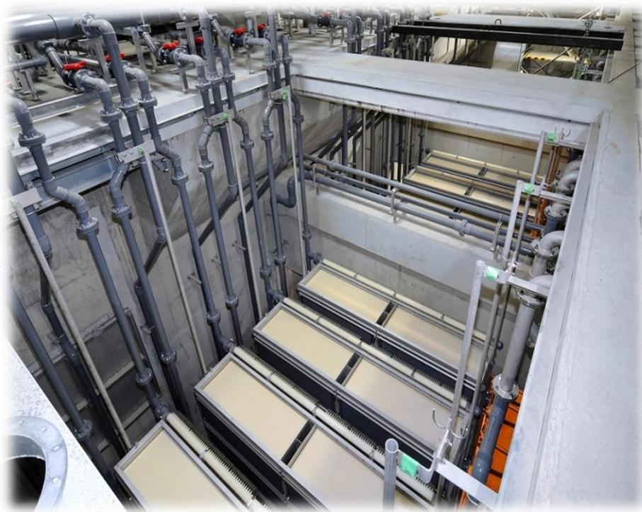
**Fig. 1.3.5.** Plate membrane reactor for N – microorganisms retention and high sludge age reaching (simultaneously cleaned using the air).
